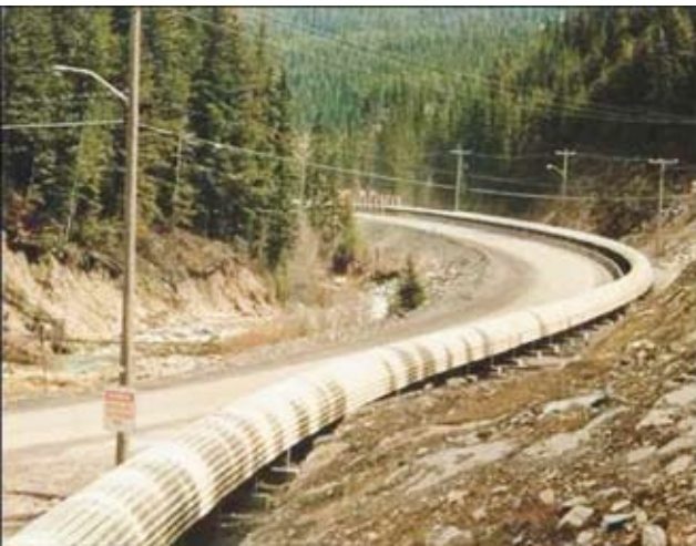
Figure 3. A horizontally-curving conveyor.
