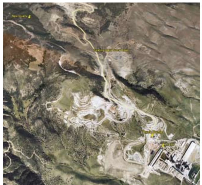
Figure 2. Lebec plant, quarry and haul road.
